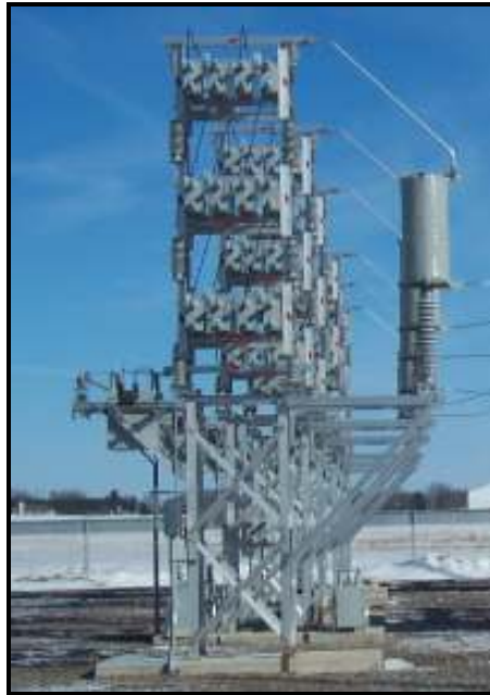
Figure 2-3. Shunt Capacitor Bank with current limiting reactor [30]
