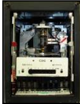
Figure 2-7. CDG16 Electromechanical earth fault relay
