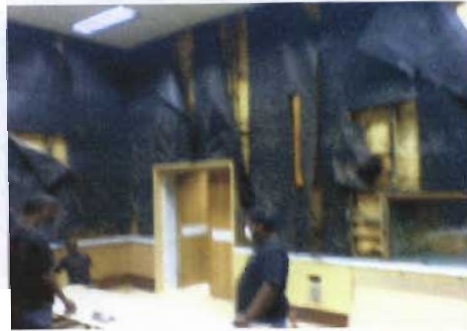
Plate 39: Refurbishment in progress at Studio
