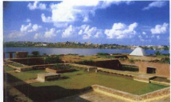
Plate 10: Planted roof gardens over
