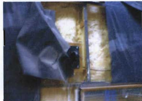
Plate 40: Fibrous Insulation Material with Fabric cover
