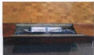
Plate 34: Raised Stage and Electrical Services access panel
