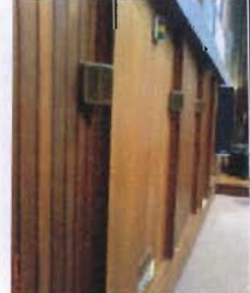
Plate 35: Angled Acoustic Panels on flanking walls
