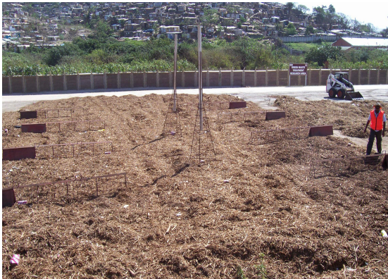
Plate 4.7: Setting out of DAT materials and filter base
