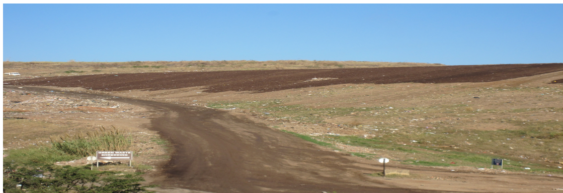
Plate 5.7: Final slope partially dressed with the compost
