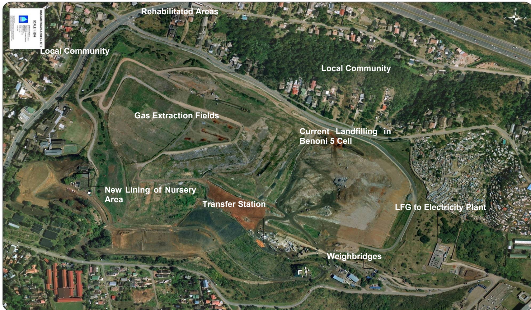
Figure 3.4: Aerial view of the Bisasar Road Landfill Site
