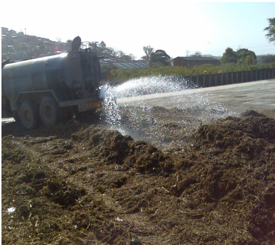
Plate 4.5: Water tanker spraying water on shredded material during construction
