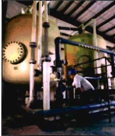
Figure 9.3: Down Flow Ion Exchange Columns [Internet] 65
