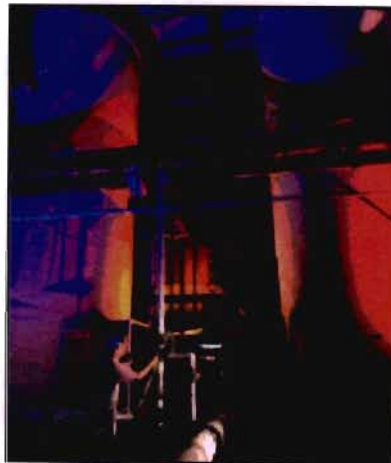
Figure 9.4: Up Flow Ion Exchange Columns [Internet] 65
