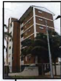
6 storey apartment block
