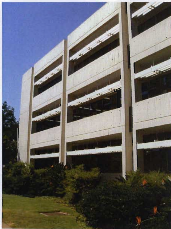
Fig 5.1.14 The 1 st year studios on the 2 nd floor. Note the north and south facing clerestories. (Source: author)
