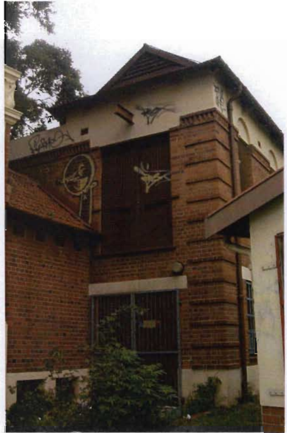
Fig 7.5.3 A historically valuable abandoned sub-station building on the site. (source: author)
