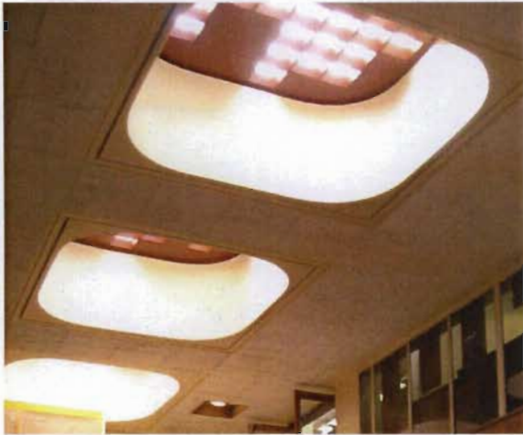
Fig 5.1.13 Skylights above the central volume – glass blocks cast in random patterns into the concrete roof slab. (Source: author)
