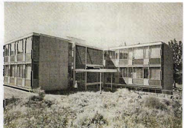
Fig 5.1.1. The original 1961 structure viewed from the North-West. Note the extensive unshaded glazing on the North façade and the blinds closed behind the glass. (SA Arch Record, June 1961, p10)
