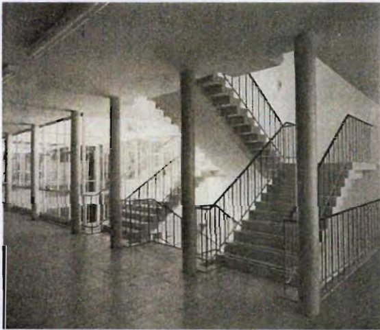
Fig 5.1.2. The main stairs, placed adjacent to the central atrium. The unusual design of the stairs is borrowed from the Bauhaus' main stair, reinforcing the design's clear allegiance to modernism. (SA Arch Record, June 1961, p12)
