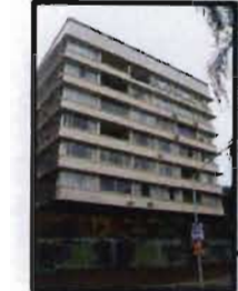
6 storey apartment block
