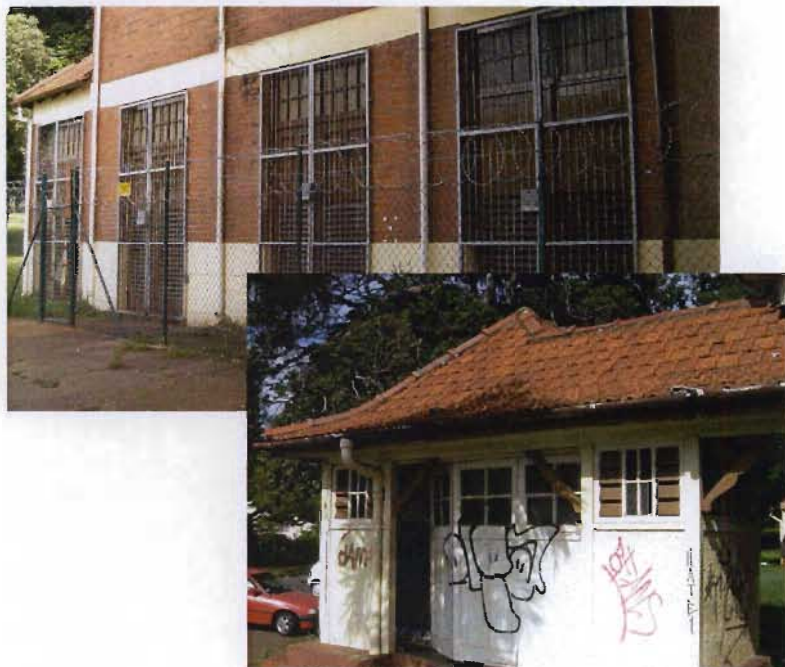
Fig 7.7.7 The terrible state of the Bulwer Park buildings (Author, 2008)
