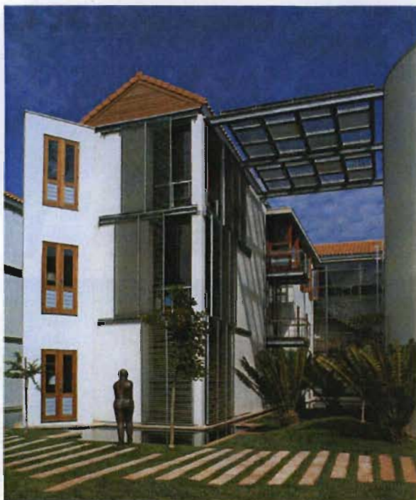
Fig 3.2.2 One of the wings specifically designed for the Judges' Chambers (Arch SA, July/Aug 2004, p12)
