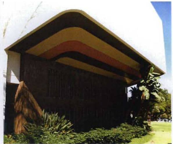
Fig 5.1.6. The back of the main lecture hall projects out on the northern facade. Note the retro paint scheme. (Source: author)
