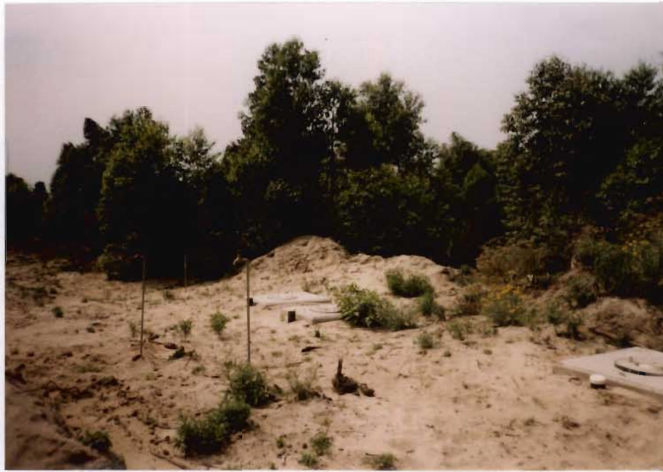
Photograph 6: The services provided include two calamite tanks (on which the owner must build their own top structure) and standpipes.
