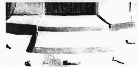
Steps to hut showing double layers and stone edging. Photo: Author:2000
