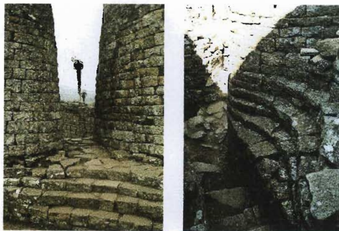
Upper; Drain constructed to bottom of Inner Wall (Author) Lower; Curved stone steps at Northeast Entry to Great Enclosure (Author)
