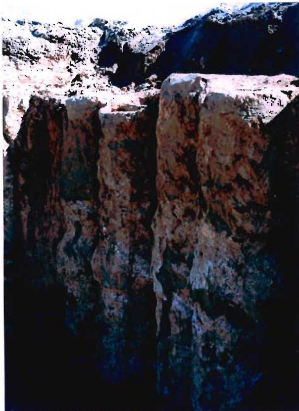
Figure 9. Appearance of excavated jet grout column showing interlock between columns. Column diameter is 600mm nominal.
