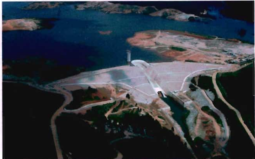
Figure 2. View of the completed dam showing inlet tower, trough spillway and outlet conduit with main embankment.
