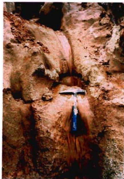
Figure 11.2. Turbid water exiting from piping erosion on the right excavation flank in granite saprolite.
