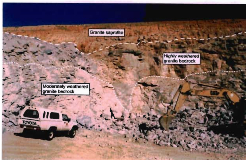
Figure 4.3. Typical weathering profile encountered at Injaka Dam site. Note the distinct lack of core stones with the very abrupt contact separating granite saprolite from highly weathered granite bedrock.
