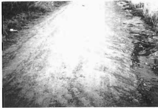
Photograph of road taken at Siphofu by the researcher.
