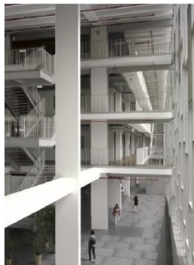
FIGURE 5.9 : open staircase links upper and lower levels adjacent to the glazed curtain wall, attracts student interactions (Source: https://www.archdaily.com/227874/ewha-womans-university-dominique-perrault-architecture - Accessed 8 November 2020)
