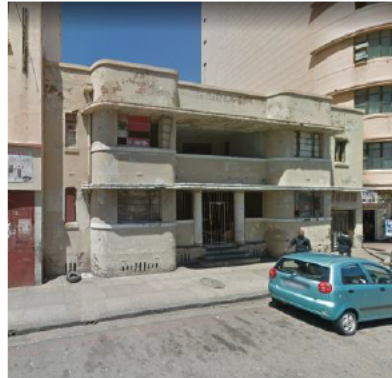
Figure 7.21: All Ameen building. (Source: Author 2020)
