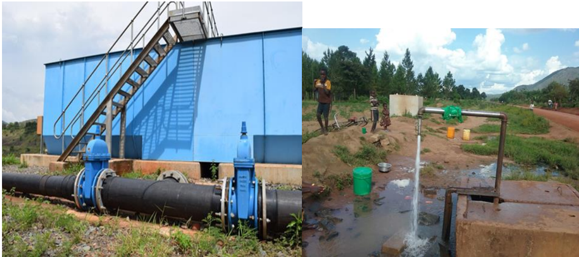
Picture 8: A Water tank and one of the water outlets at Nyakabale Village
