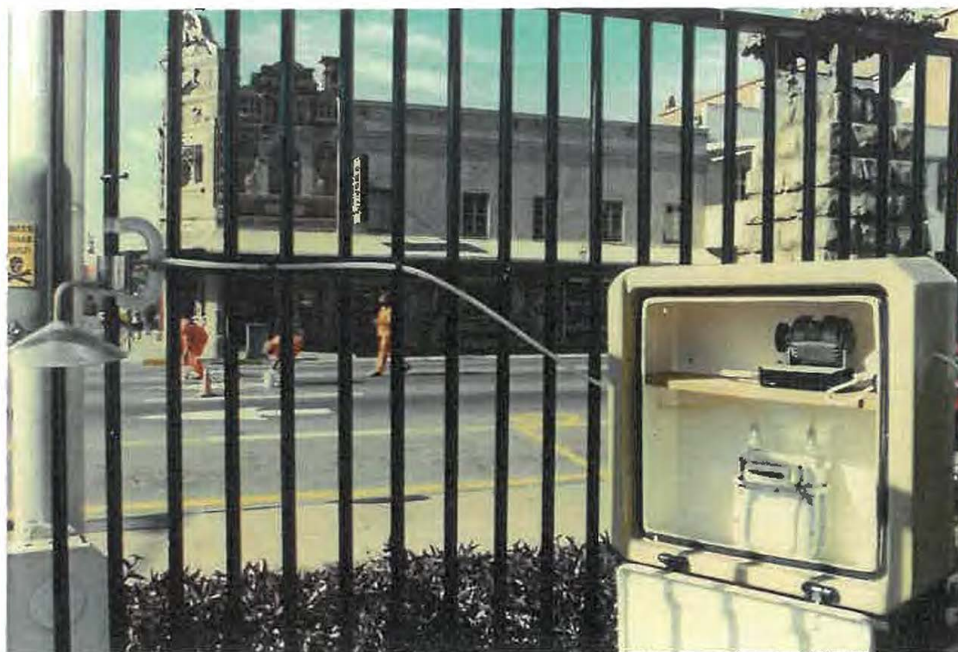
Figure 12: Filter unit and housing adjacent to monitoring laboratory. Inlet funnel, gas meter and suction pump are visible while gas washing bottles are absent as only smoke is being measured. Longmarket Street is in the background.
