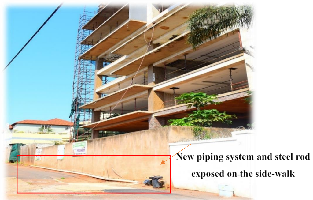
Plate 4. 4 Exposure to incomplete pipelines and steel rods which are hazardous to pedestrians (Author, 2018)
