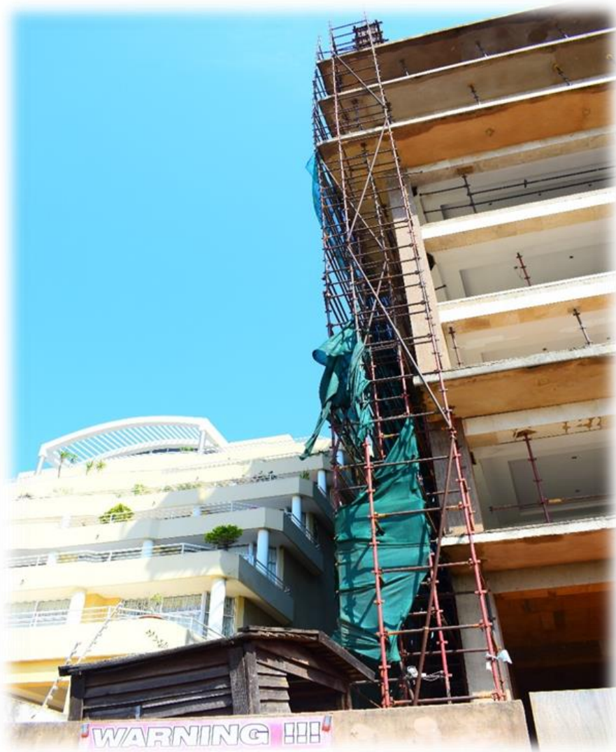
Plate 4. 6 Scaffolding on premises for approximately four years (Author, 2018)
