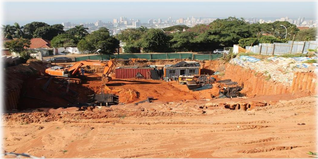
Figure 2. 1 Residents uninformed of construction at 615 Stephen Dlamini Road (Walford, 2017)
