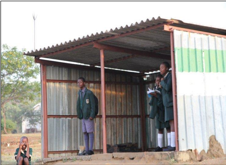
Figure 7.2: Shade Constructed by Mimosa in Zvishavane
