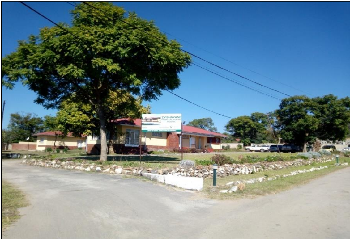
Figure 7.5: A Section of Zvishavane District Hospital Renovated by Mimosa
