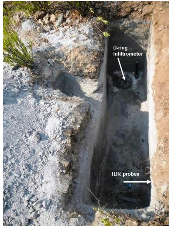
Figure 3-3: Double-Ring infiltrometer used for material characterisation at a sampling site with TDR placement indicated on the side(TSF).
