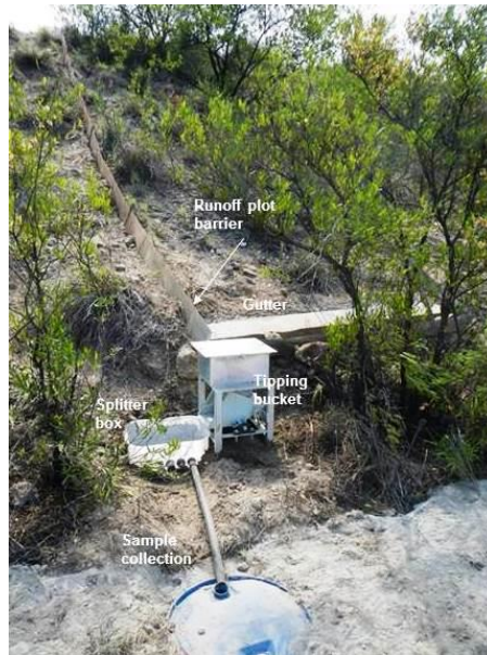
Figure 3-8: Runoff plot with a tipping bucket and event logger as installed on the Tailings Storage Facility, with barriers on the side to ensure that only runoff inside the test area would be measured.
