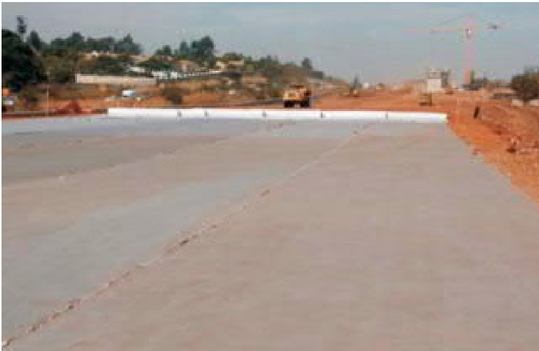
Figure 1-2: Use of Geotextiles in Reinforced Platform over Sinkhole Prone Areas along the Gautrain Route in Gauteng, South Africa (Gewanlal 2009)
