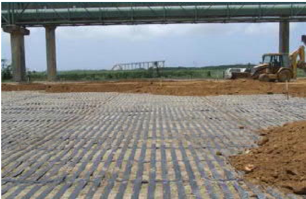
Figure 2-8: Basal Reinforcement over Soft Soils to Increase the Bearing Capacity of the Subsoils for the Construction of Warehouses at the Valley Terminal in Richards Bay (Maccaferri 2010)
