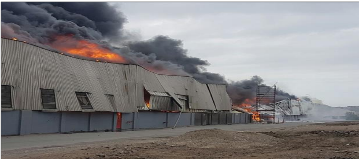
Figure 2.4: Durban Bayhead Warehouse – fire
