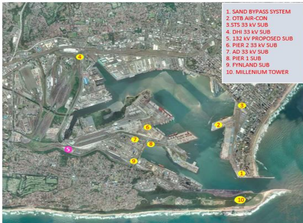
Figure 3-2: Geographically dispersed electrical substations monitored on the PoD's SCADA system [44]
