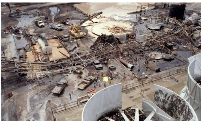
Figure 2.4 ARCO Channelview Compressor Explosion
