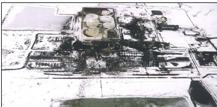
Figure 2.5 Fertilizer Plant in Port Neal Explosion
