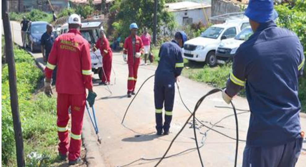
Figure 2.2 eThekweni Revenue Protection Services personnel work tirelessly to disconnect illegally connected electrical wires. SOURCE: Phoenix Sun (2016).
