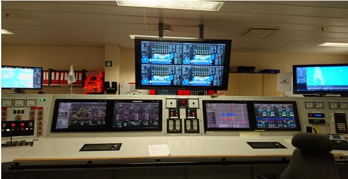
Figure 5 Engine Control Room of the Viking Grace, Source: Author
