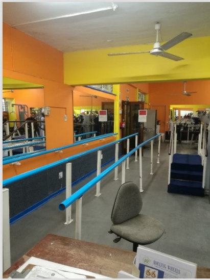
Figure 6.2.4.4.1 – Rehabilitation Gym toilet (source: Author)
