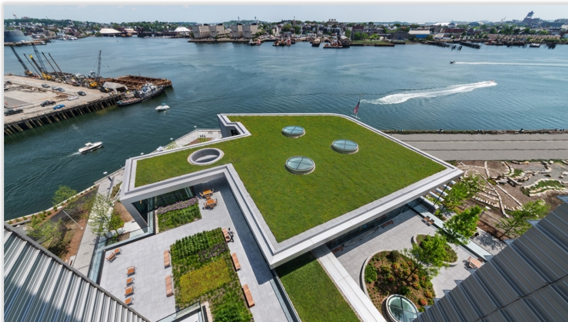
Figure 5.2.2.2.1 –The Roof garden as seen from the upper floors (Source: www.archdaily.com )
