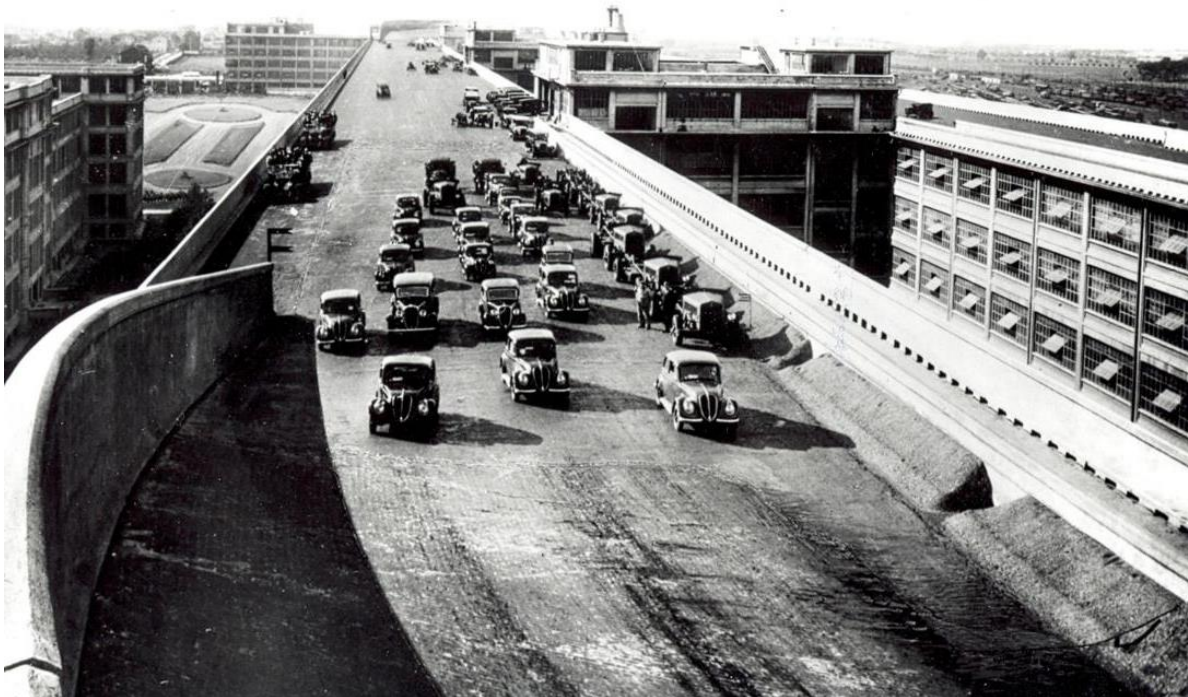
Figure 5.3.4 A race track in the sky (Fiat Group, 2014). The racetrack on the roof level of the existing building.
