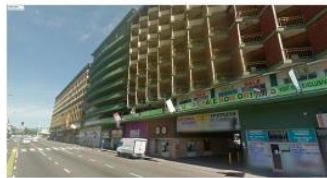
Perforated brick facade
