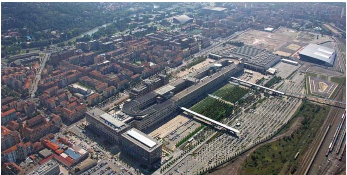
Figure 5.3.5: (top) Building within the urban context of Turin (Google Earth, 2018). Figure 5.3.6: (bottom) A race track in the sky (Fiat Group, 2014). Aerial view of the factory in relationship to the railway line and the River Po.
