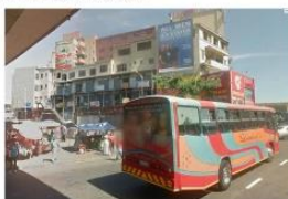
Building from main access road
