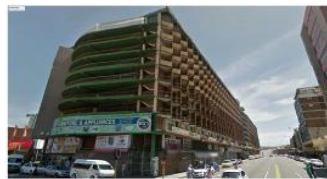
South East facade
