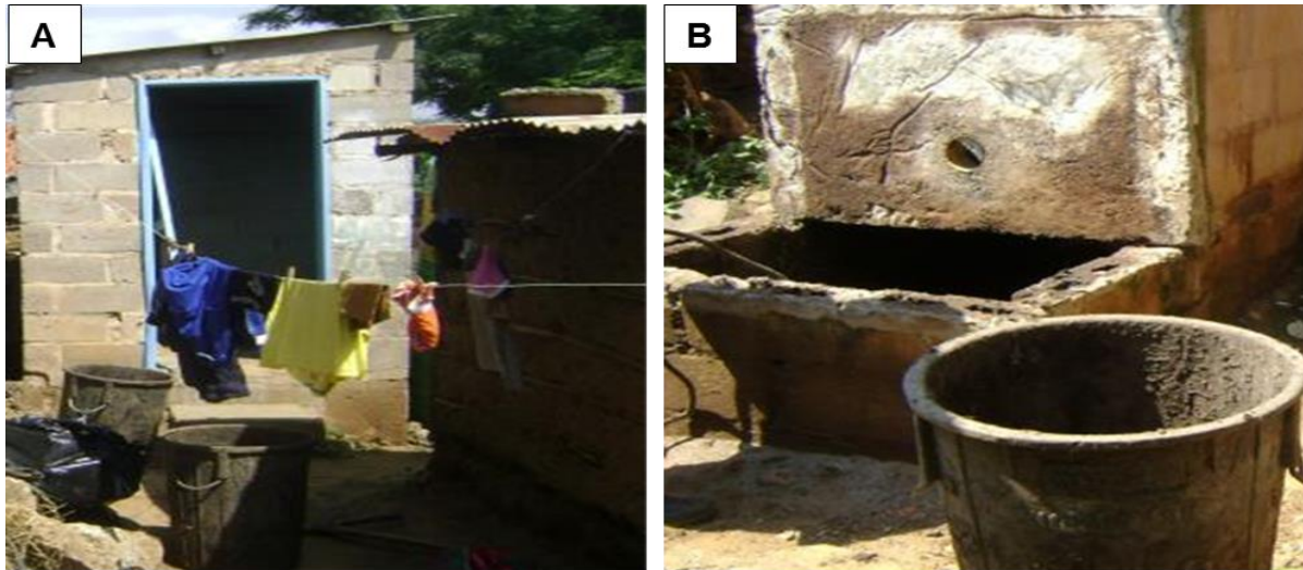
Figure 1 Ventilated improved pit latrine (VIP) structure. (A) Entrance to VIP, (B) area where pit latrine fecal sludge is collected when the pit is full.
