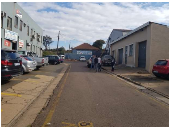
FIGURE 90 – CONTEXTUAL EXTERIOR VIEW
