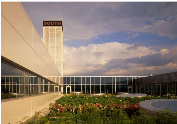
Figure 79 - Exterior finishes (Curtain Wall)
