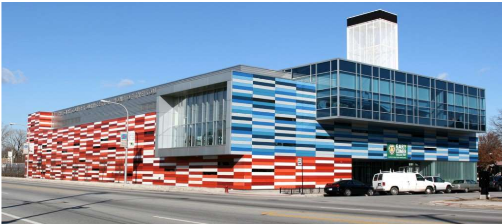
Figure 71 - South views of the Gary Comer Youth Center Available at: https://www.archdaily.com/ [Accessed 28 June 2018].
