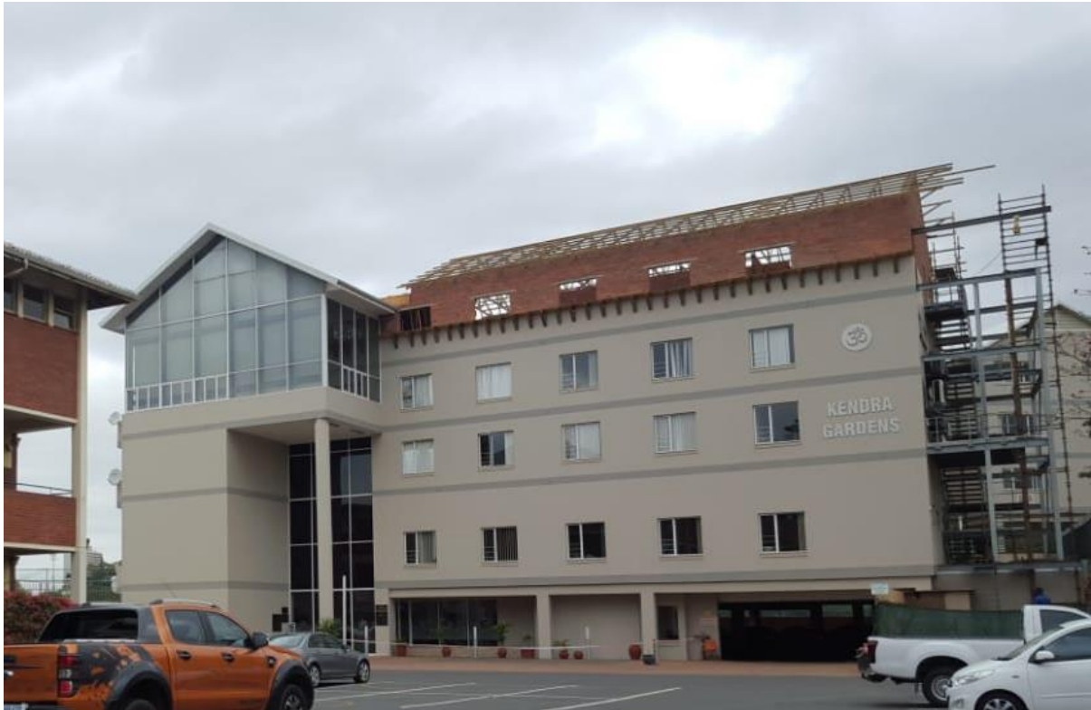
Figure 75 – North View of The Kendra Gardens Retirement Home
