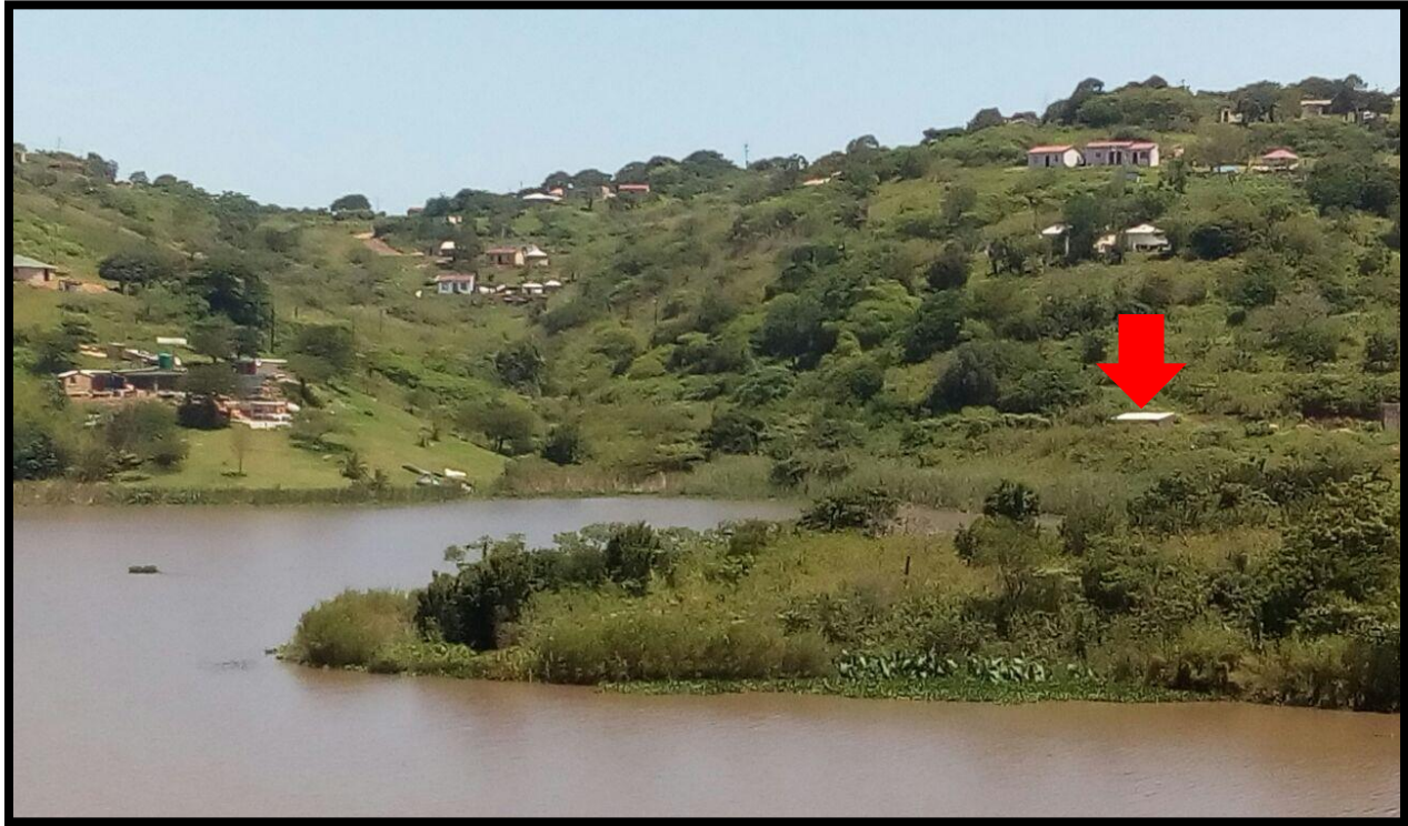
Figure 6.12: Image showing Housing or Settlement Developments occurring near UMnini Dam
