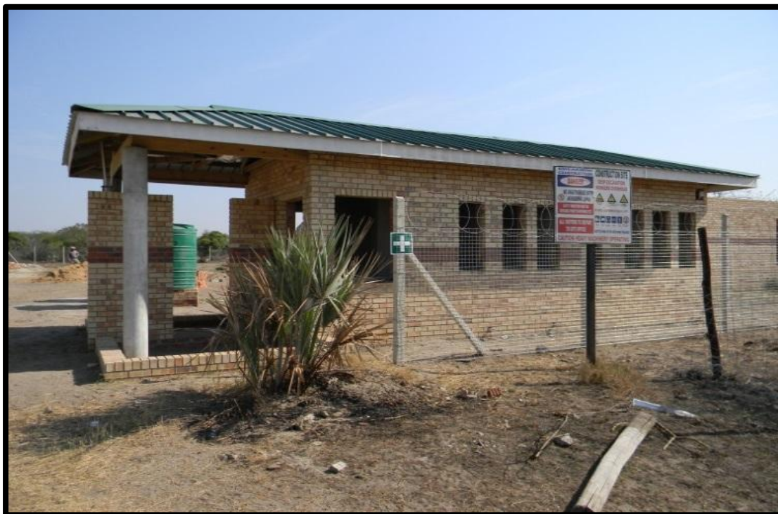
Figure 9: Local Clinic that is under construction at ward 16, Mthembu M., September 2016
