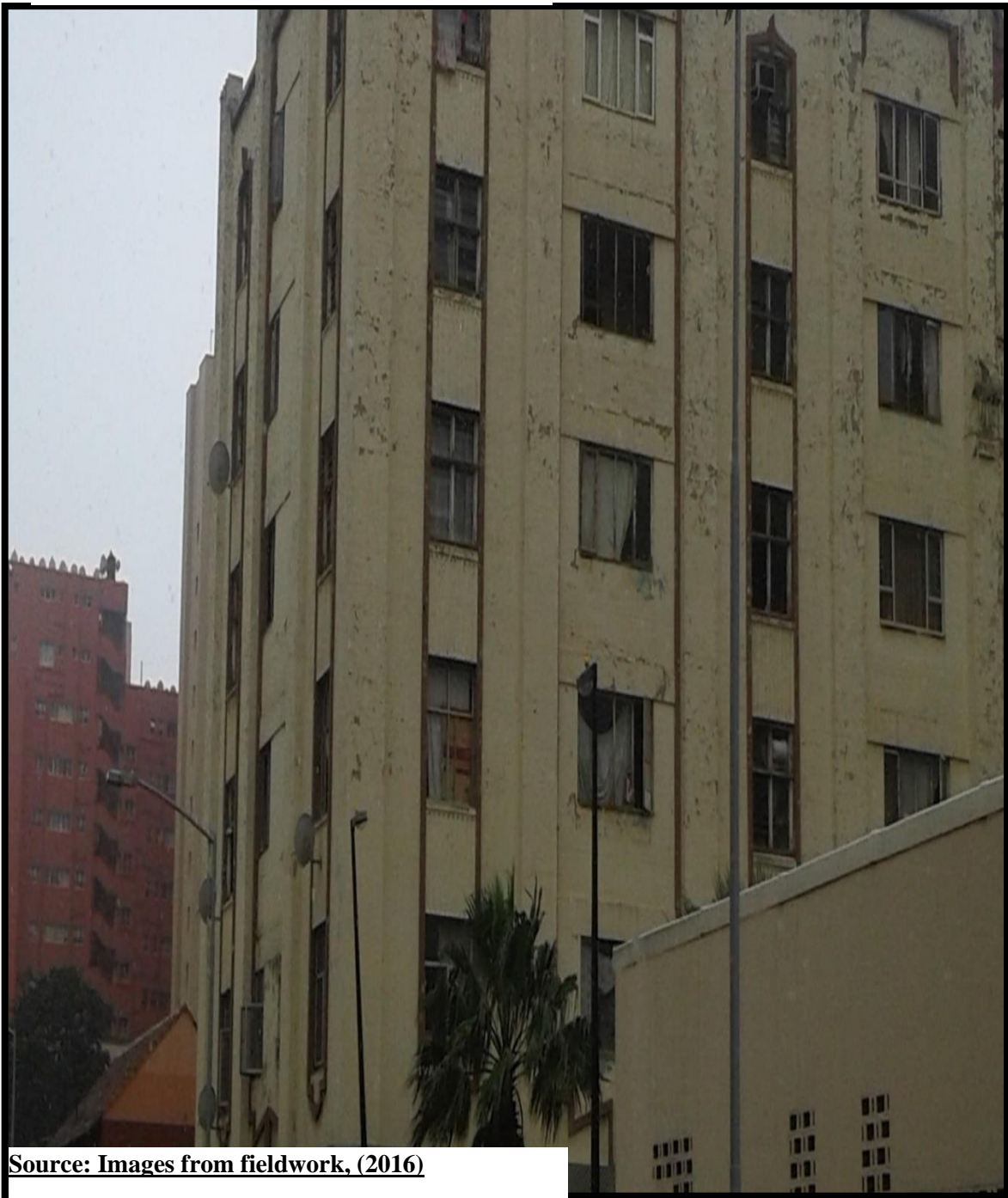
Image 6. 1: Paint peeling-off the walls
