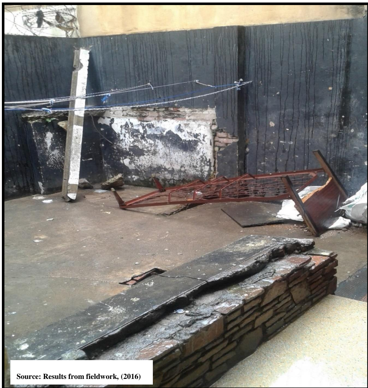
Image 6.2: Lack of maintenance
