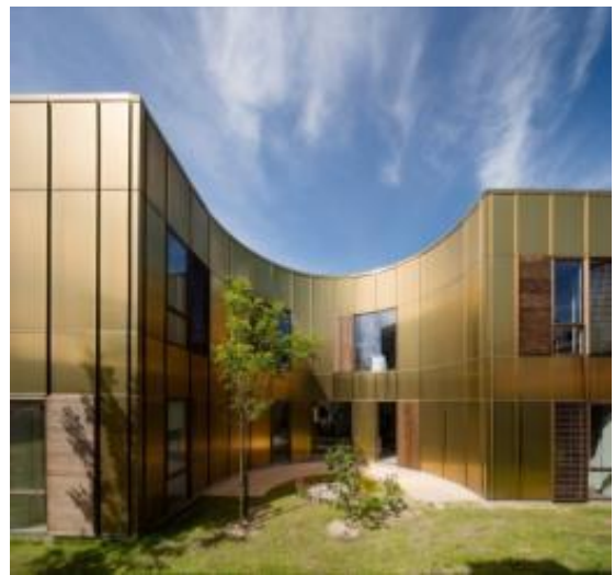
Figure 50 view of courtyard
