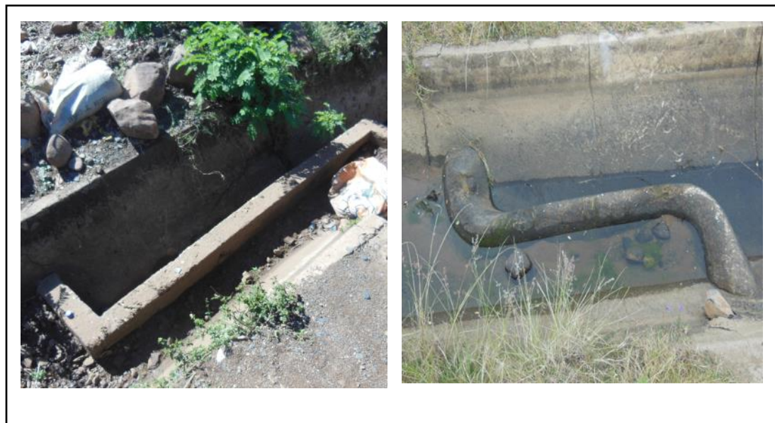
Figure 3.8 Debris clogged discharge weirs in MRIS
