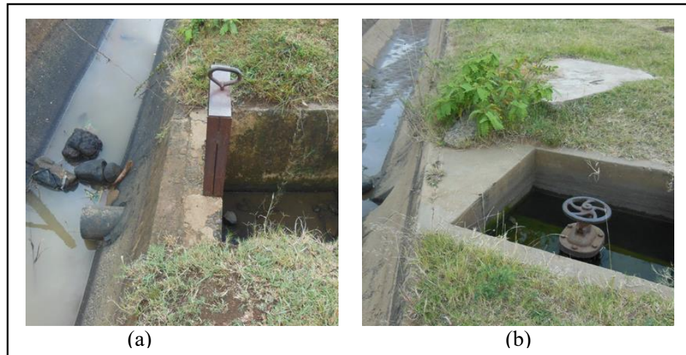
Figure 3.7 (a) Typical sluice at abstraction point and (b) typical valve at the abstraction point
