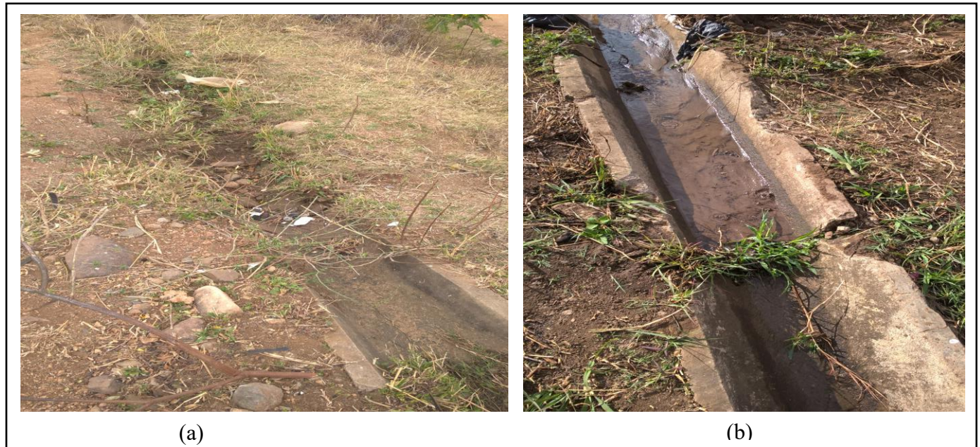
Figure 5.6 (a) Silted canal and (b) cracks and failed concrete lining
