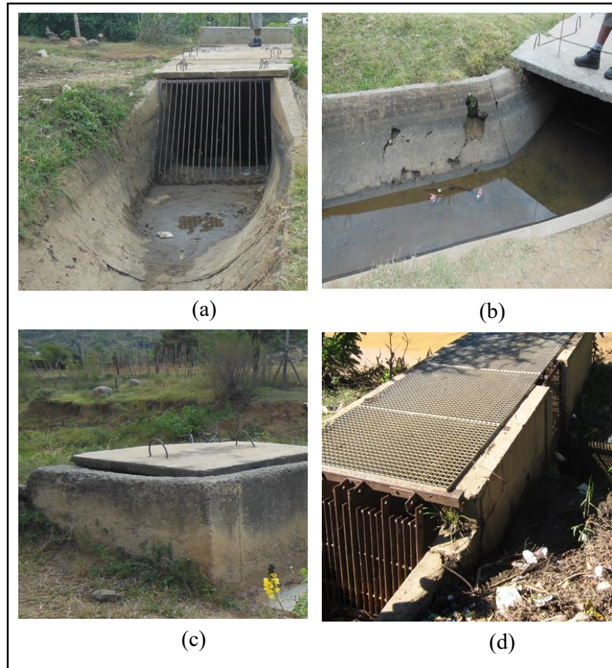
Figure 3.6 (a) The siphon inlet, (b) siphon outlet (c) the scouring chambers at head end and (d) the scouring chambers at the tail end
