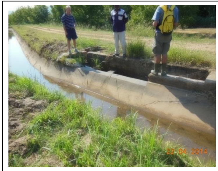
Figure 3.9 Side spillway located along the 25 km canal ( Element Consulting Engineers, 2014 )
