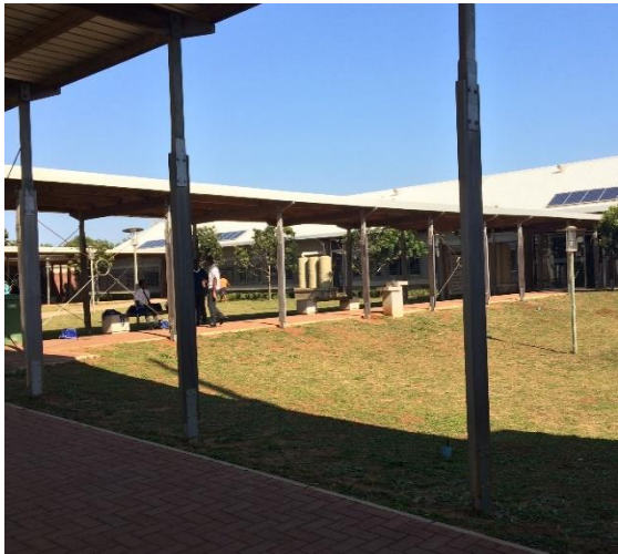
FIGURE 4.1.4.2: Covered Walkways with Seating. Solar panels on the roof; SOURCE: Author
