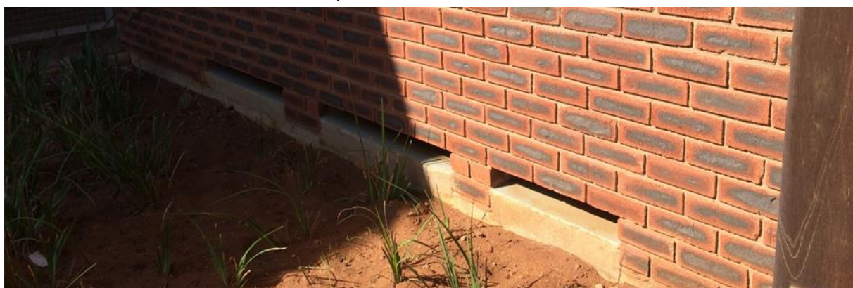
FIGURE 4.1.4.7: Under Counter Ventilation Openings in Toilets; SOURCE: Author
