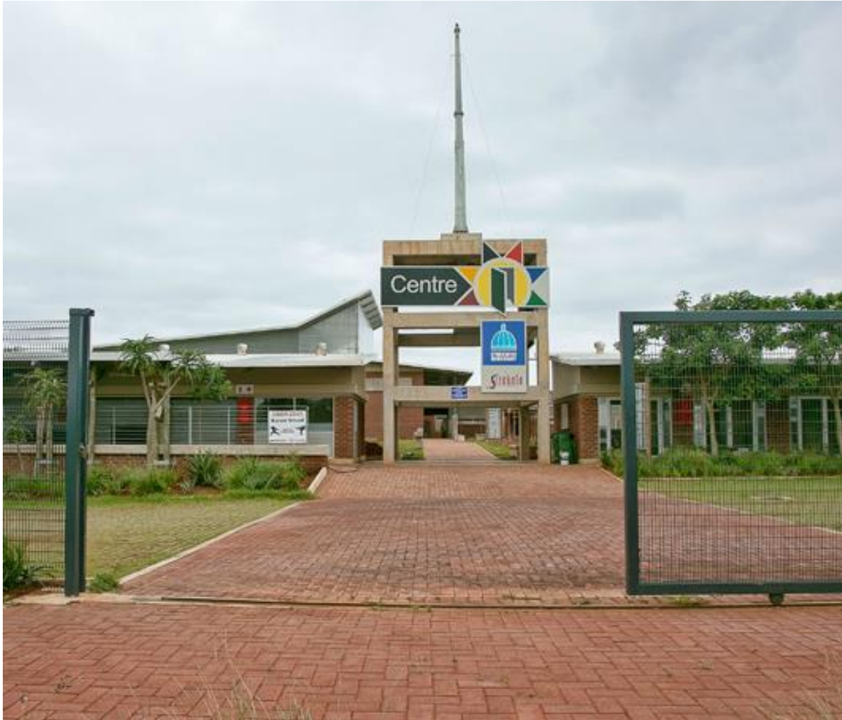
FIGURE 4.1.1: Entrance to uMnini Thusong Centre; SOURCE: eThekweni Municipality, Accessed August 2017 < http://www.durban.gov.za/City_Services/engineering%20unit/City%20Architects/Documents/ThusongCentre.pdf >
