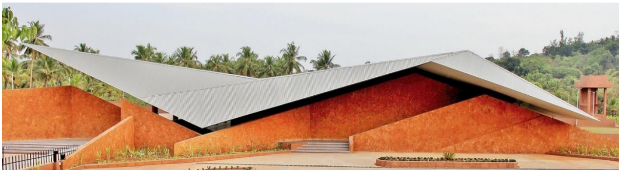
FIGURE 3.3.3.1: Walls mimicking the landscape and roof mimicking suspended rain clouds. SOURCE: Archdaily, Accessed November 2017 < https://www.archdaily.com/798500/valpoi-busstand-and-community-hall-rahul-deshpande-and-associates >.
