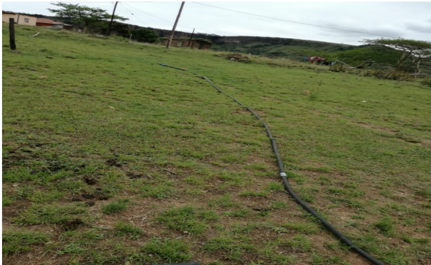
Figure 4: Pipes Connected to Well
