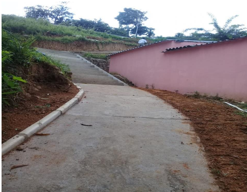
Pic 6: Passage constructed under the EPWP: Taken by the researcher.
