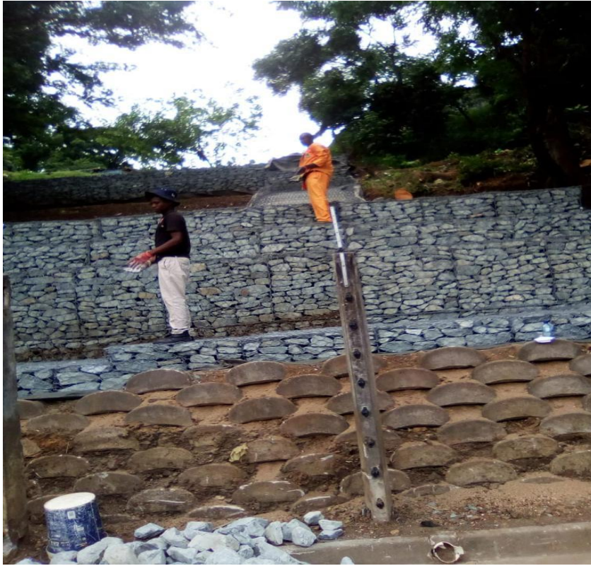
Figure 3: Worker with no uniform: Taken by the researcher.
