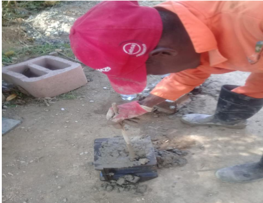
Pic 5: A worker mixing cement. Taken by the researcher
