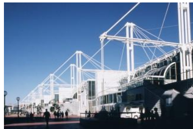
Figure 150: Building by Cox Architects located in the Sydney Waterfront
