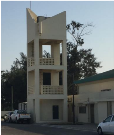
Figure 89: The water tower. Source: Author
