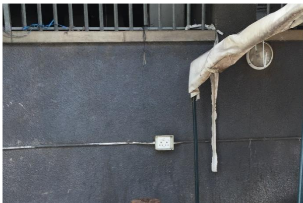
Figure 71: Plug points located throughout the market.
