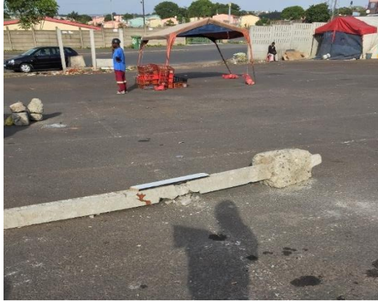
Figure 80: Part of the concrete fence that has been broken to get access to the high grade steel inside the concrete Source: Author
