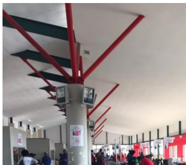
Figure 94: Indicating the lighting system within the fish market.
