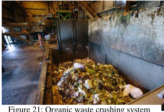
Figure 21: Organic waste crushing system Source: https://www.sustainabilitymatters.net.au
