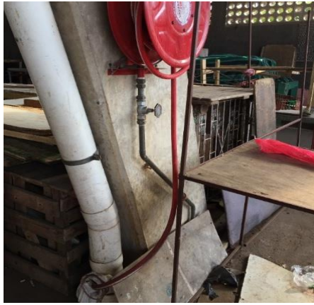
Figure 63: Leaking fire hose reel that is simply connected into the municipal storm water pipes Source: Author
