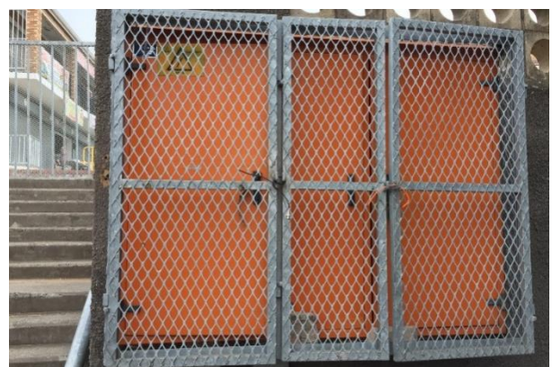
Figure 72: Electrical switchgear located at the entrance
