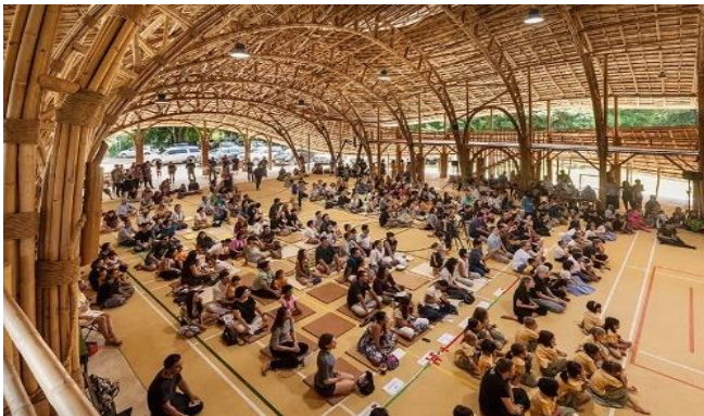
Figure 154: Image showing the magnificent bamboo structure that spans over 18m.
