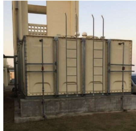
Figure 90: The storage tanks on the ground Source Author
