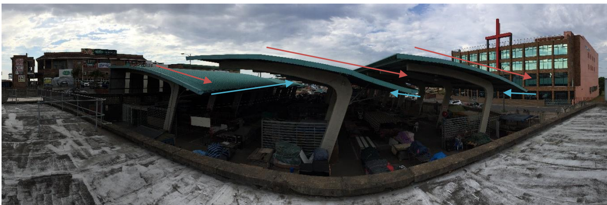
Figure 66: Image of the roof layout, as well as how and where the water is collected in the gutters. Source: Author
