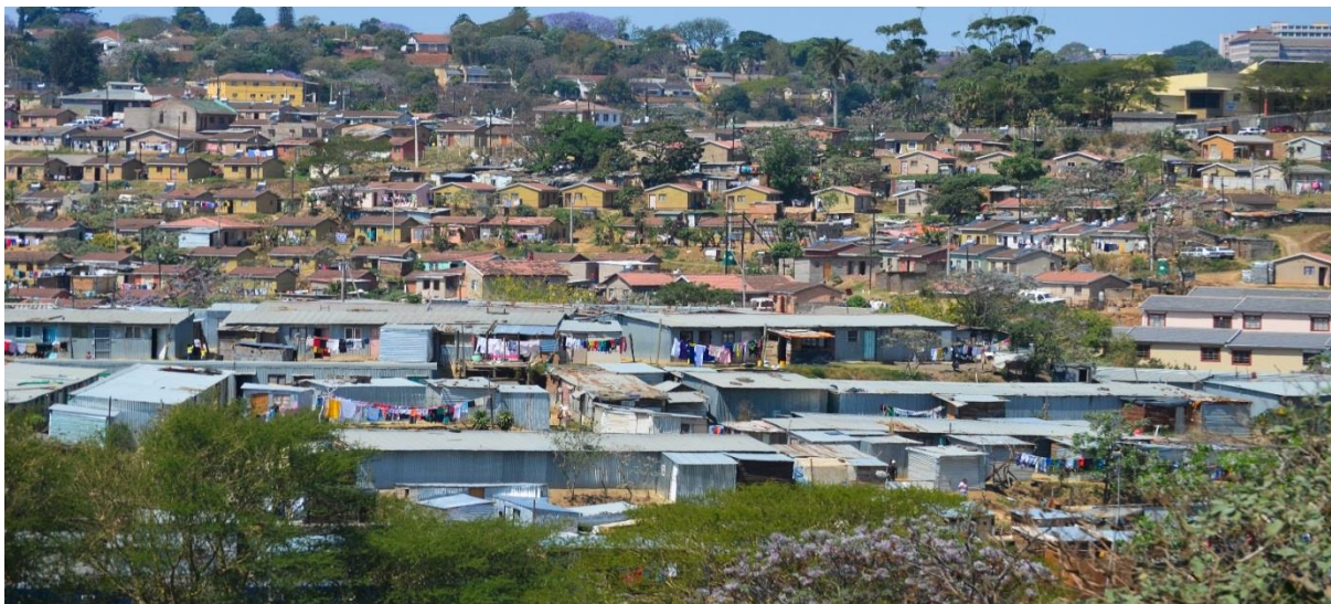
Figure 2: illustration of Cato Crest area with formal and informal settlements existing beside each other
