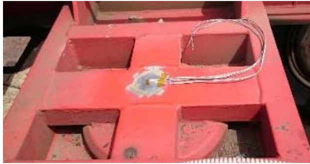
Figure 5.2: Rosette gauge installed at top of kingpin support
