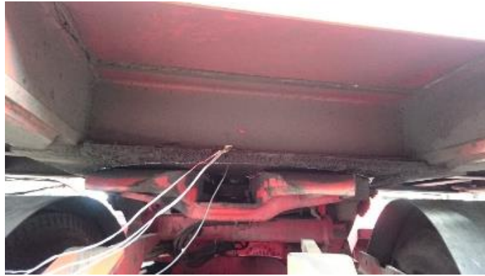
Figure 5.22: Rosette gauge installed at kingpin supporting structural member. (Direct access to the kingpin was not possible with the top plate of the trailer).
