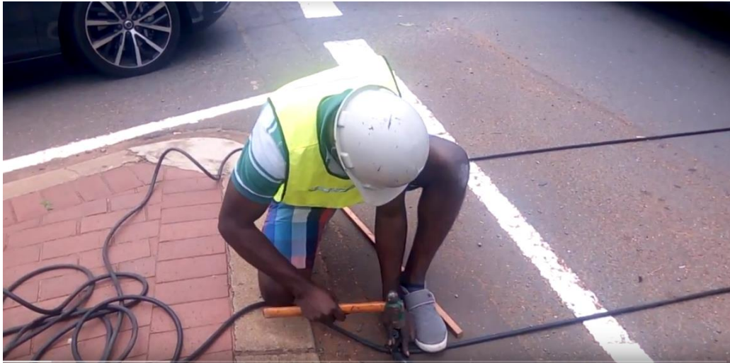
Figure 3.7: Pneumatic tube laying process at the circulating roadway at Douglas roundabout
