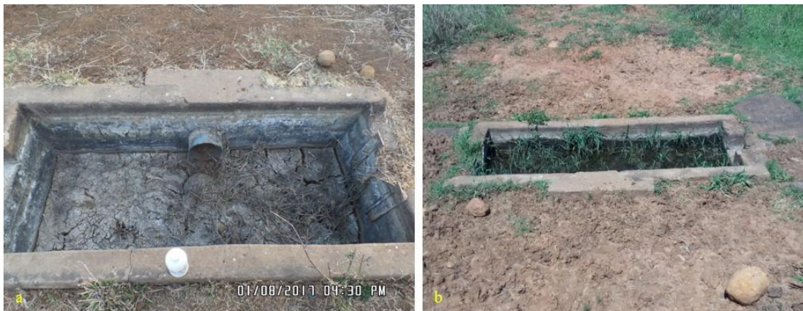
Figure 6.1: Splitter to cell 5 and 6 clogged with debris and dense algal growth (a) winter; (b) summer
