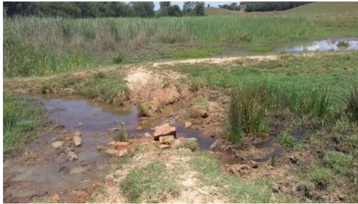
Figure 6.6: Degraded berm between cell 1 and 2 due to trampling by animals
