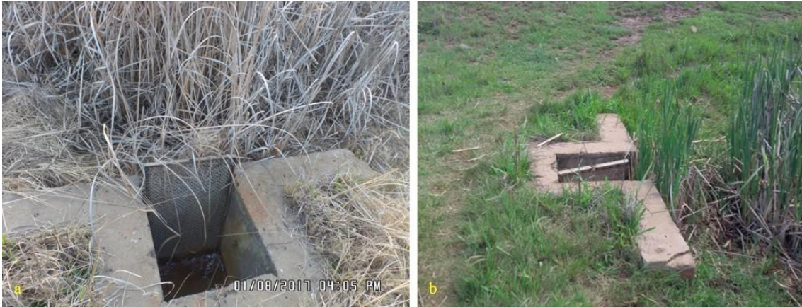
Figure 6.3: Splitter to sub-surface pipe from cell 4 which connects to the splitter to cell 5 and 6, (a) upper part shows cell 4, lower part shows splitter; (b) left side shows splitter; right side shows cell 4
