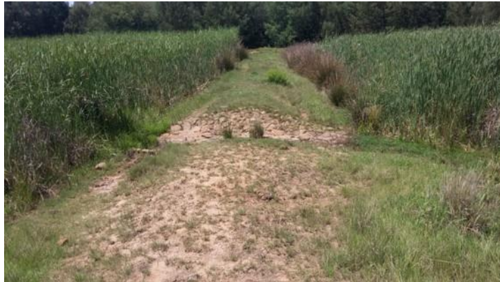
Figure 6.2: Two cells separated by a berm with dense growth of Typha
