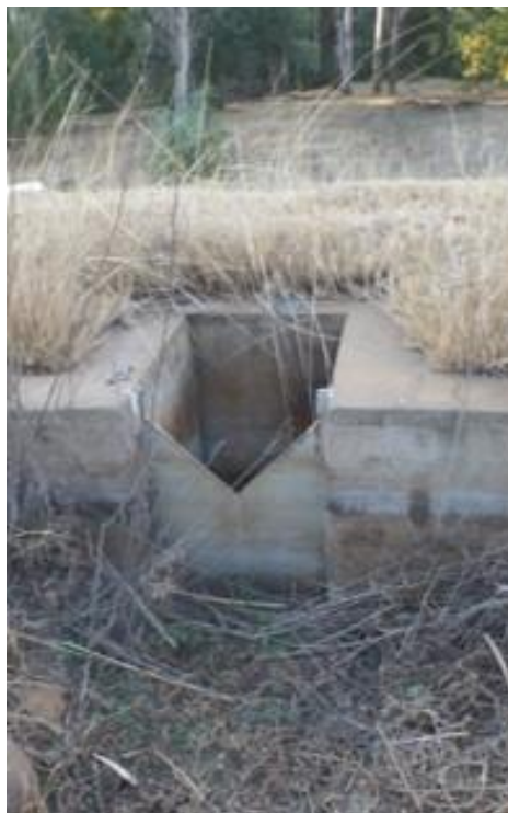
Figure 7.4: Mechanism leading water out of the wetland (from cell 10) and into the river. This part of the wetland has not been functional for a significant amount of time
