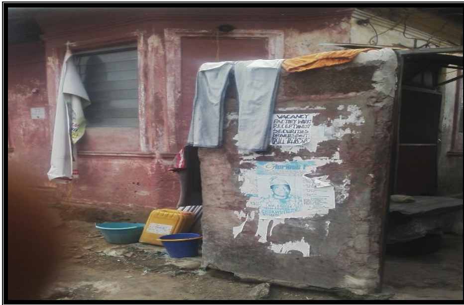
Plate 7.4: Poor quality housing occupied by the poor in the inner city
