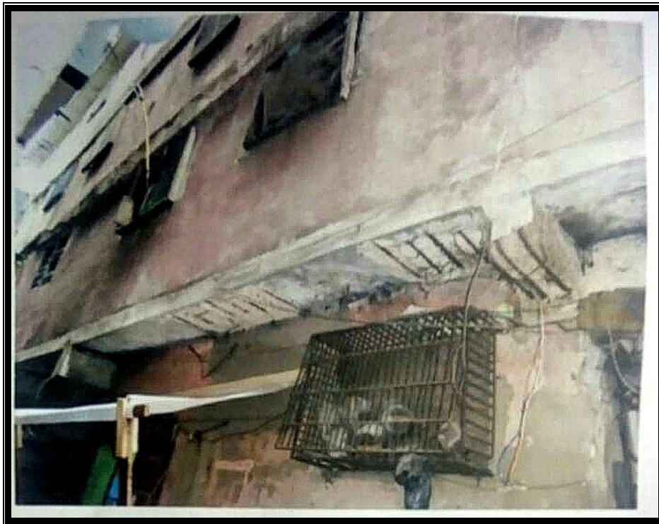
Plate 7.1: Dilapidated housing in Obalende
