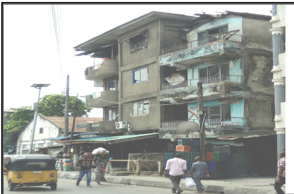
Plate 7.2: Dilapidated building in Obalende
