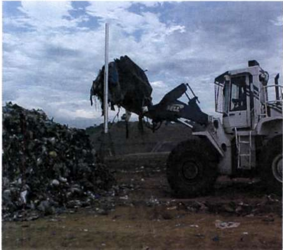
Figure 4.7 A front-end loader placing the wet mixture
