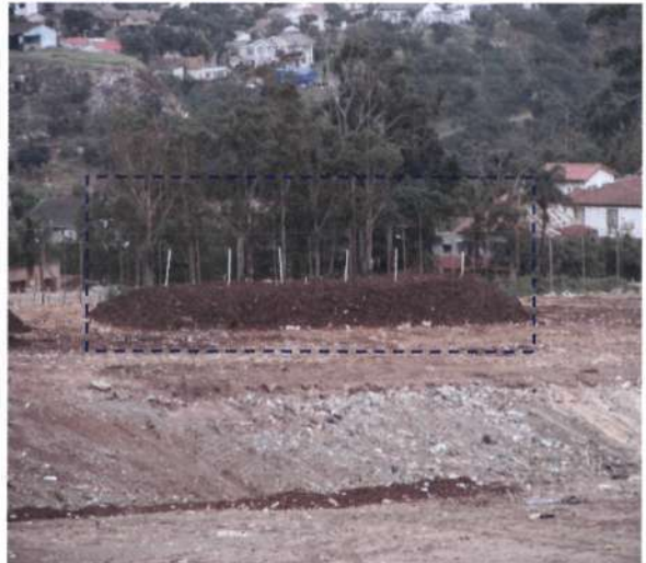
Figure 4.8 A completed windrow
