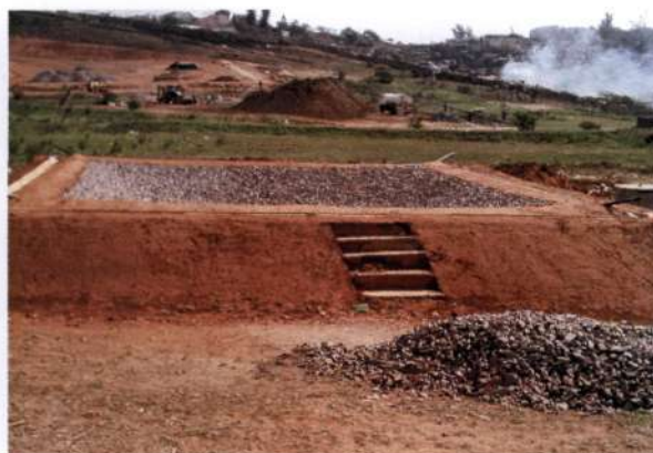
Figure 6.5 A completed cells
