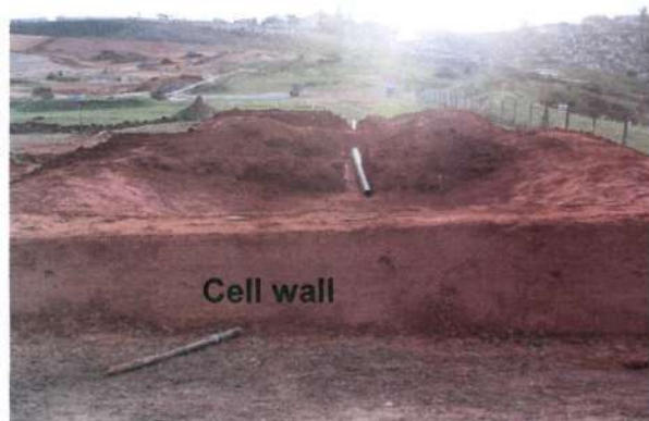
Figure 6.2 Construction of cell walls
