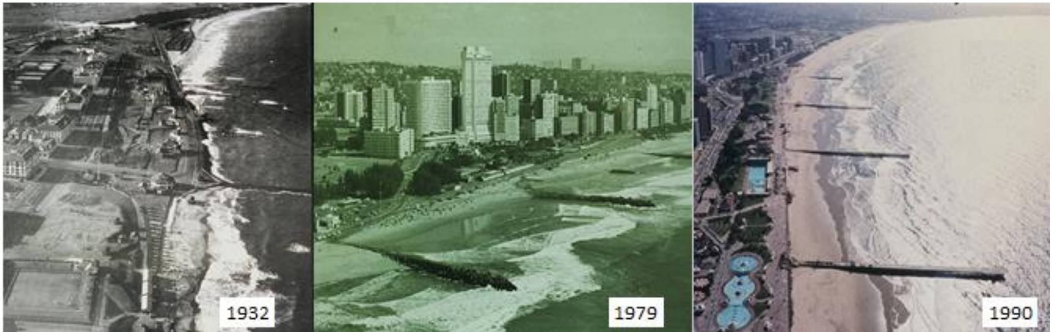
Figure 1-2: Types of groyne systems implemented over the years at Durban beach front in trying to solve coastal erosion (Barnett, 2011)
