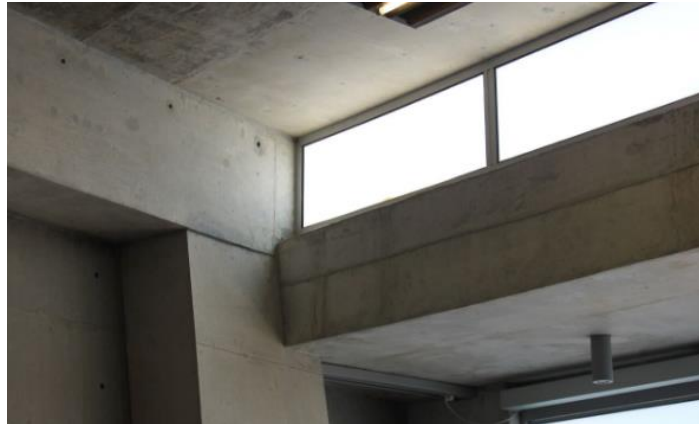
Fig 6.14 Clearstory windows for natural sunshine and play of solid and void (Source by Author)
