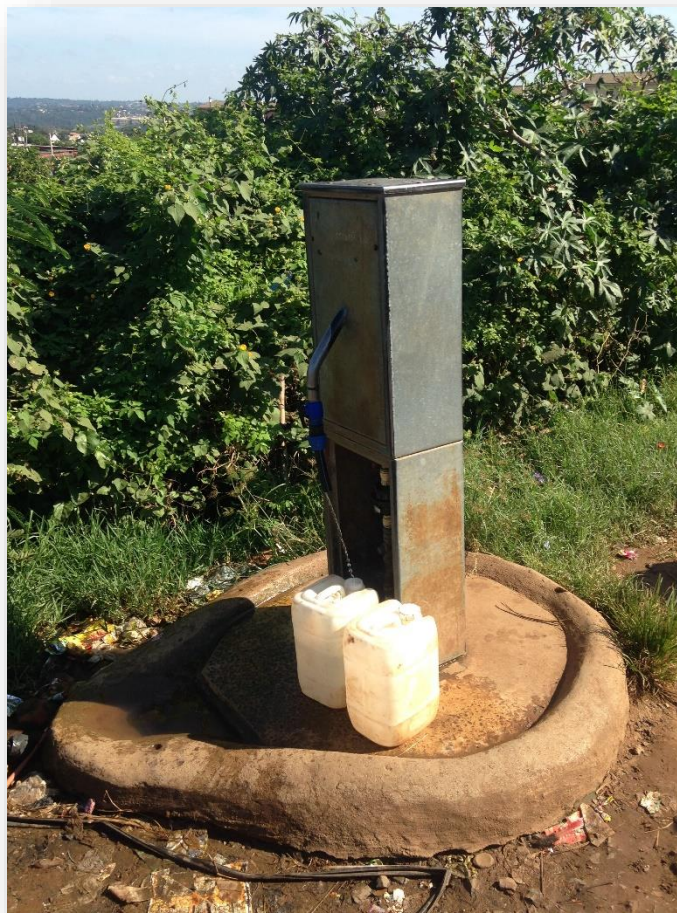
Figure 15: Communal standpipe with low flow of water in Cato Crest upgraded informal settlement.
