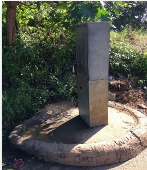
Figure 10: Communal Standpipe in Cato Crest providing safe drinking water.
