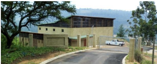
Figure 161 Community Hall at Entrance to Village. IY
