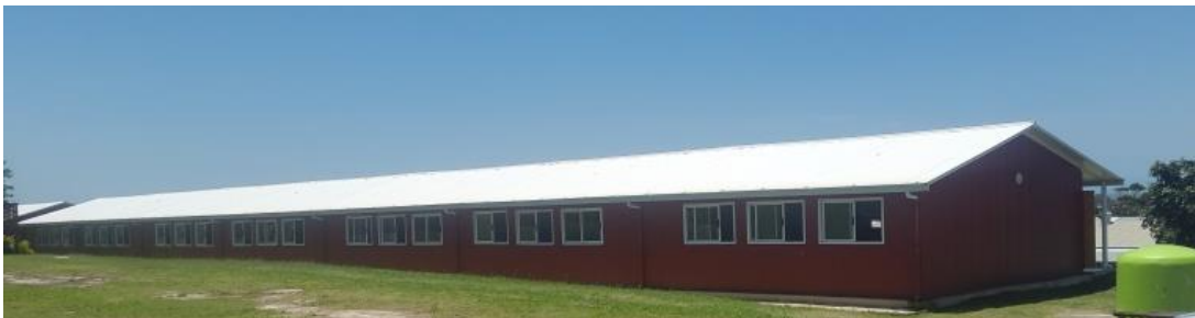
Figure 118 Village school building. LIV
