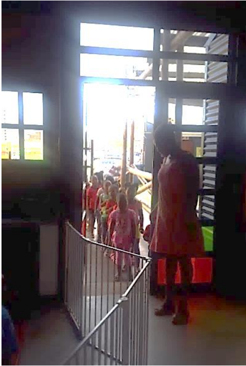
Figure 61 Interior exterior connection through 5 double doors. Q ECD
