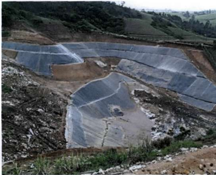
Figure 2.1: The lining of the Shongweni Landfill Site.
