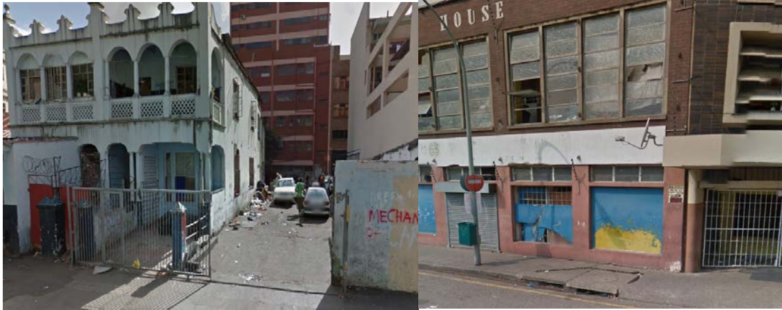
Figure 9 & 10: The exterior of two dilapidated buildings in the Durban inner city (Author, 2015).
