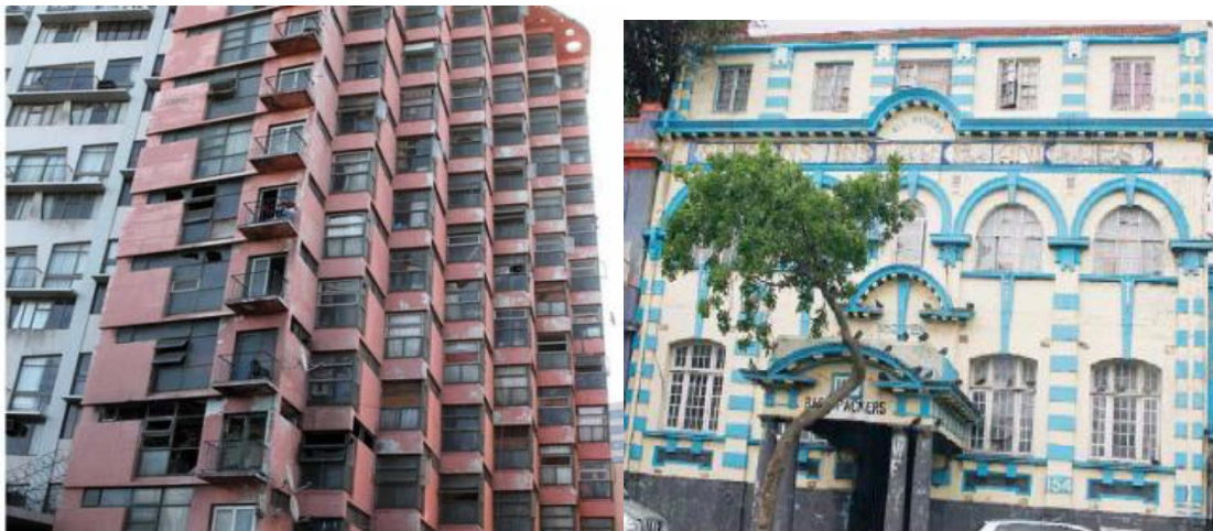
Figure 15 & 16: Two of the dilapidated buildings purchased by the Municipality for Social Housing (EThekweni Municipality, 2015).
