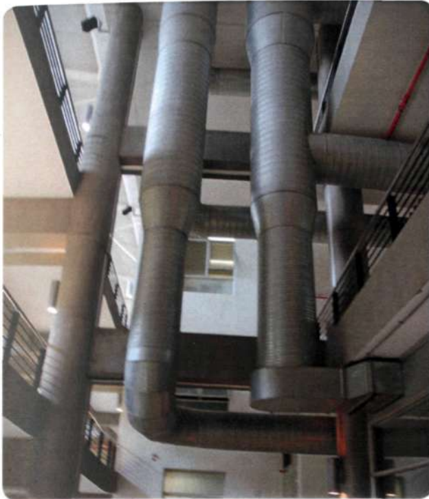
iii.5.23: The large air-con ducts which have been exposed and service the studios, creating a mechanical cross ventilation through the studios.
