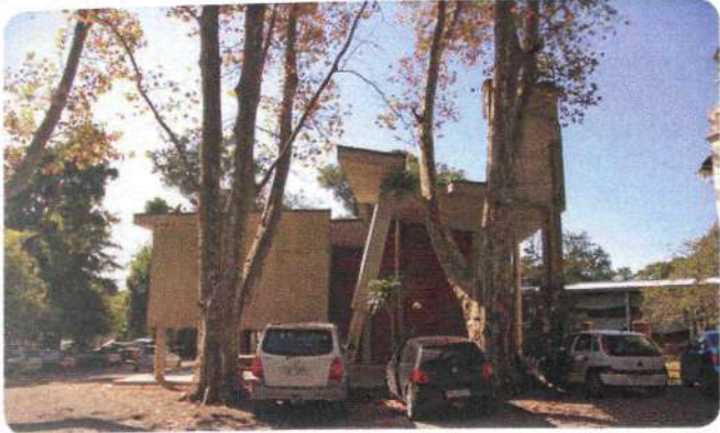
ill.4.05: The poetic use of concrete shown in the creation of form
