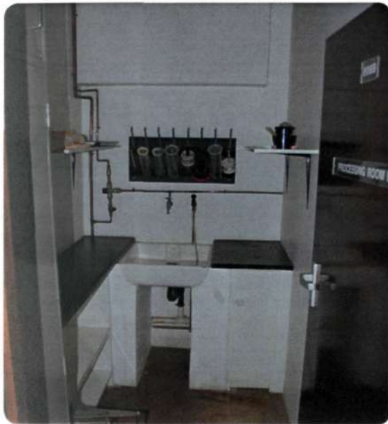
iii.5.04: A processing room in the WOSA dark room. Requires separate drainage for disposal of chemicals
