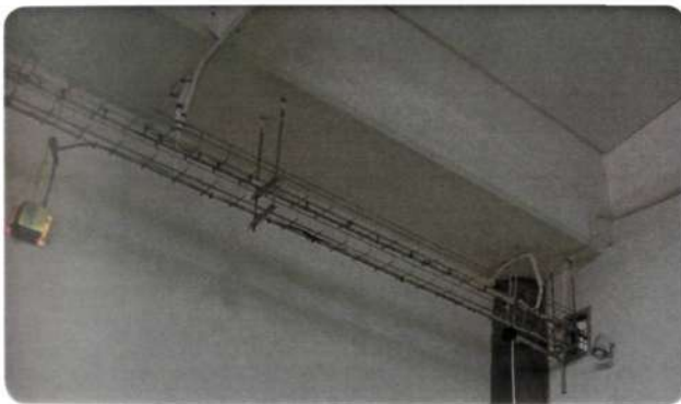
iii.5.24: The cabling system which has been employed throughout the school, continuing with the industrial concept by exposing all the "nuts and bolts" of the school.
