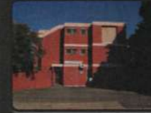
Topex N24 for the site The building is now entered from the other entrance, and therefore the Clarence Rd elevation has no interaction with the road, resulting in a dead space.
