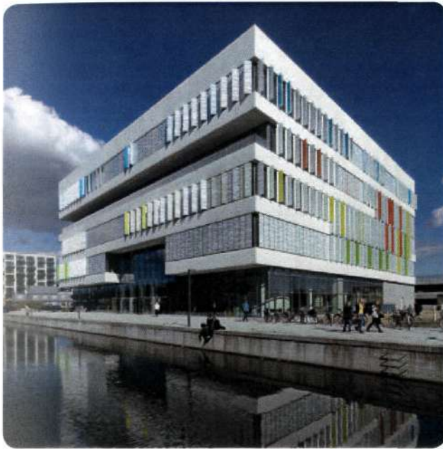
ill.4.38: A view of the school from across the canal, showing the vertical glass louvres deep floor plates.
