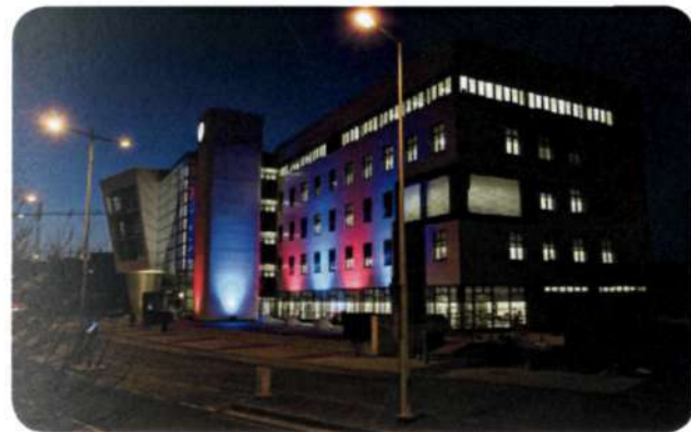
ill.4.26 Exterior view from the road
