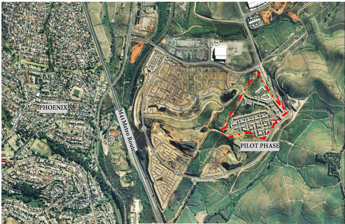
Figure 49. Image illustrating Cornubia Phase 1A: Housing, June 2016. Source: Google Earth
