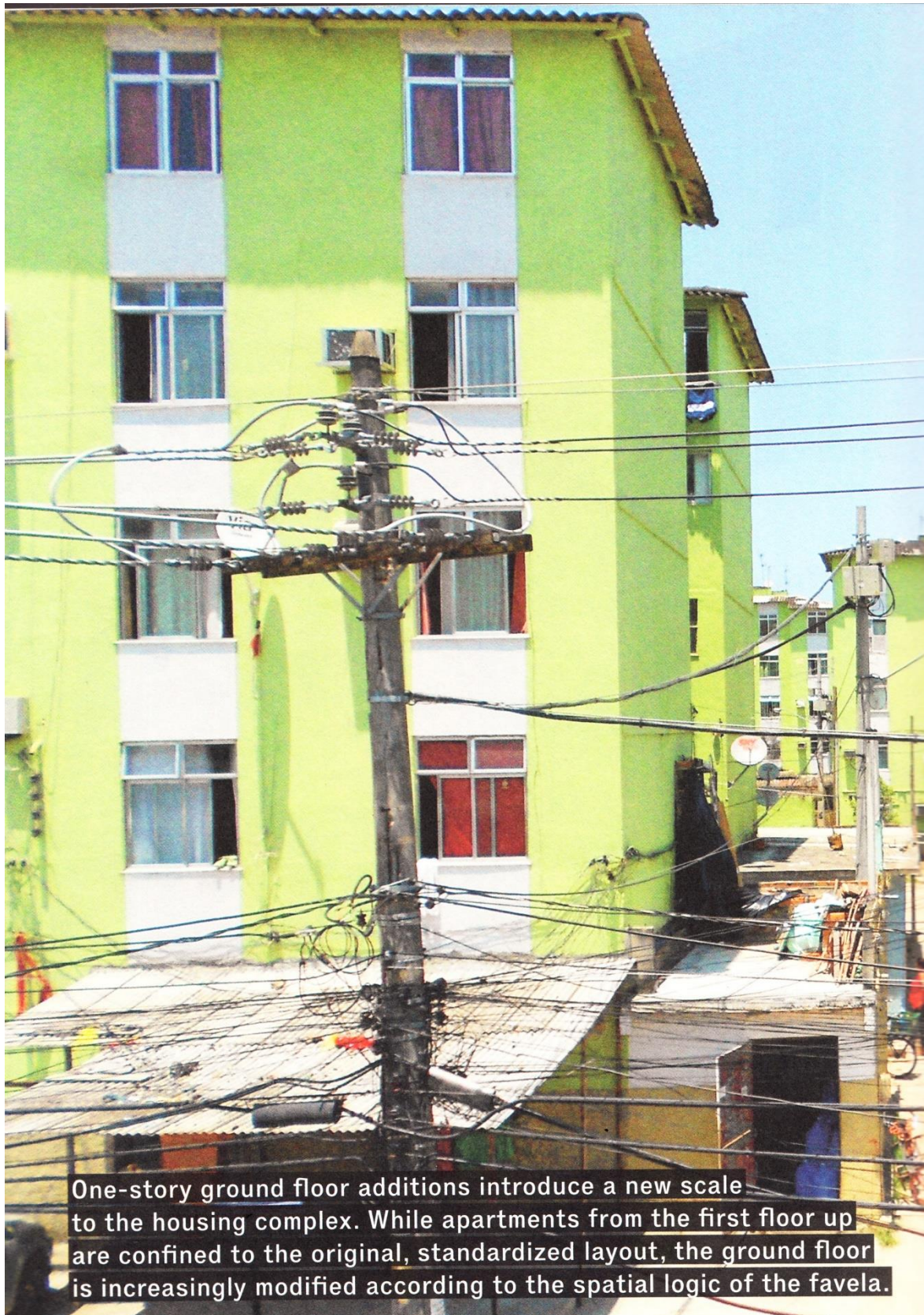
Figure 22. Image showing modernist, multi-storey residential units, constructed in the Cidade de Deus. Source: Source: Angeli and Hehl, 2013.
