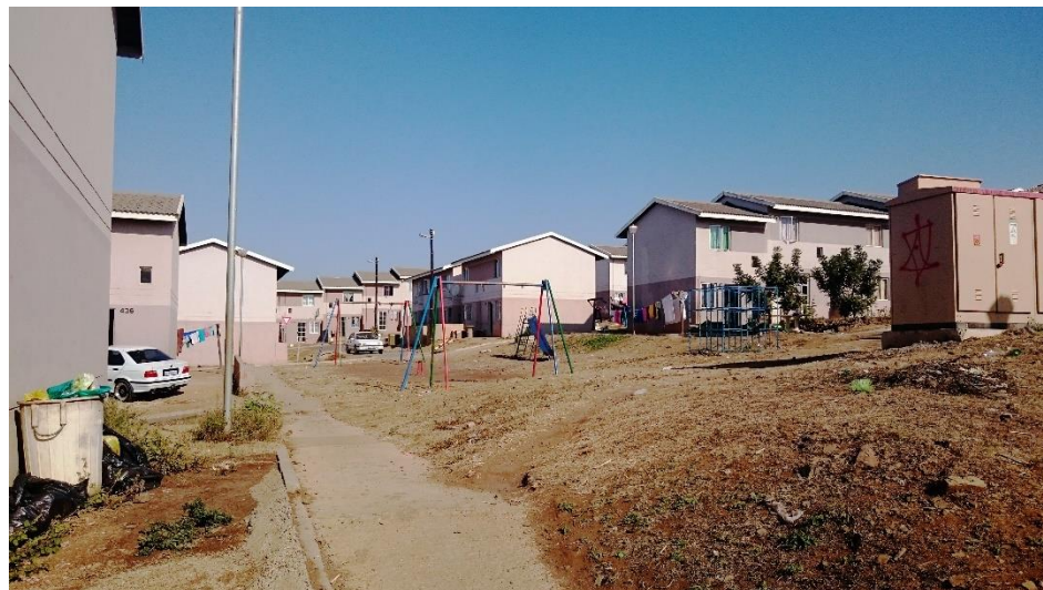
Figure 70. Image showing allocated public space – courtyards – another dead zone. This example has blank walls and service ends of houses looking onto it. This indicates poor surveillance and an underutilisation of space. Source: Author, 2016
