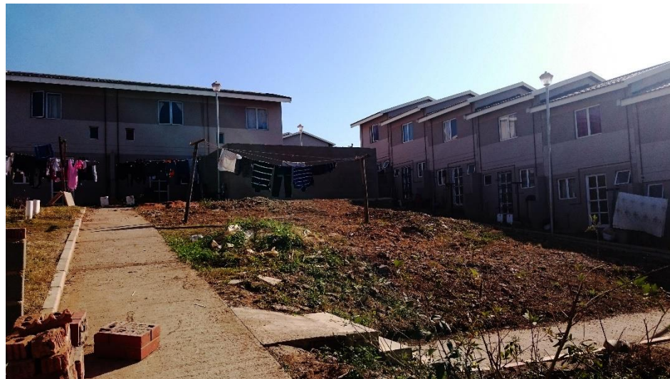
Figure 69. Image showing allocated public space – courtyards – dead zone with service end of houses – kitchen, bathrooms looking onto it. Source: Author, 2016
